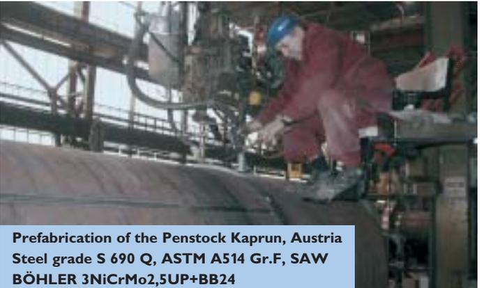
**Prefabrication of the Penstock Kaprun, Austria
